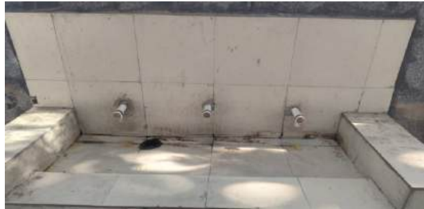
(The condition of the water facility.)
