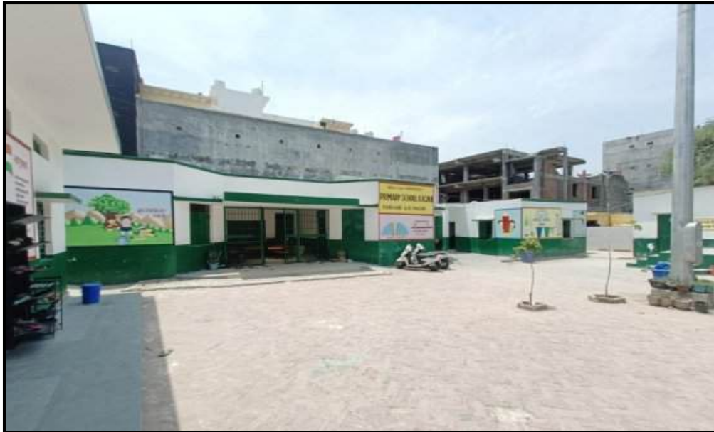
School building with baked brick walls/stone walls and roof top with slab or wooden/iron girders or tile.
